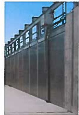
Photo 2. Fixed panel screen used during a dewatered intake project.
